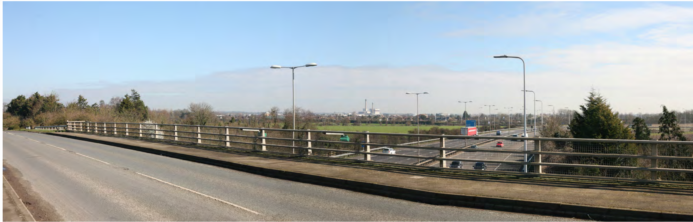
Representative Viewpoint 7, Lake End Road Bridge - Existing View
