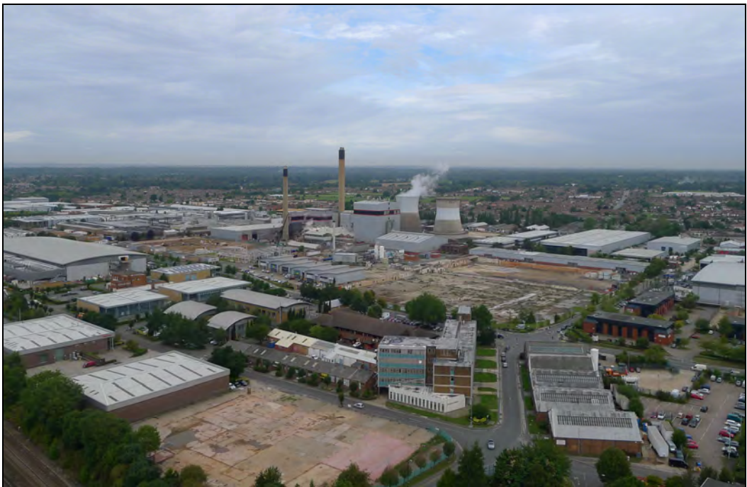
Figure 4-8 Aerial View of the SHP site from the Southeast looking in a Northwest Direction (Date taken: 19 September 2013)
