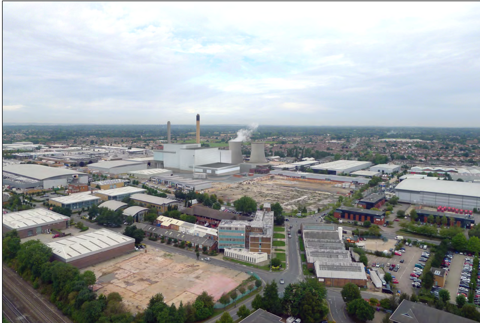
Figure 5-5 Illustrative Aerial Photomontage of the Proposed Development, viewed from the Southeast looking Northwest
